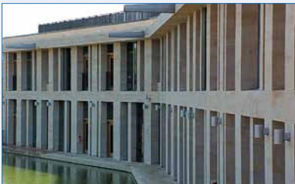
Thanks to integrated control and regulation via KNX, in this project the following reductions in energy consumption were possible: 78 % due to use of natural ventilation, 50 % due to regulation of underfloor heating in 16 zones, 60 – 70 % due to constant light regulation and additional presence sensors, 40 – 60 % energy saved in total compared to a conventional school building
